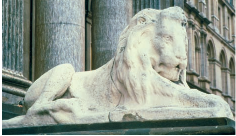
Figure 6 This stone lion sits outside Leeds Town Hall in England. It was damaged by acid precipitation.
